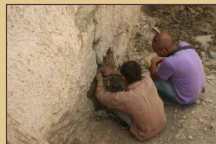
Cracks on the south eastern wall are stitched using umbu (tamarisk) and mud mortar
