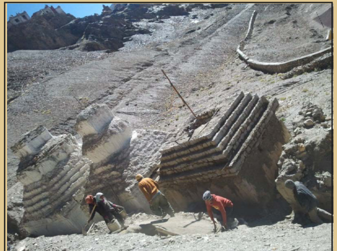
Reconstructing the four steps (pangrim) of the collapsed chorten prior to the recreation of the pungpa
