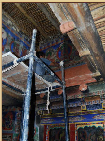
Minimal intervention to preserve the wall paintings was carried out which included consolidating delaminated layers of paint, grouting major cracks in the painted walls and cleaning the original paintings of the skylight
