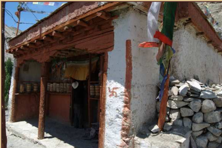
Load on the roof is reduced by removing additional layers added over the years. Proper drainage slopes and spouts were provided and the mud roof relaid
