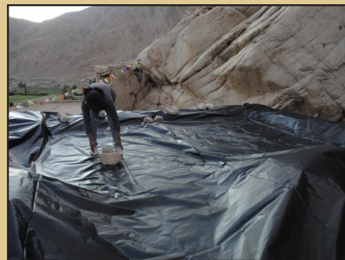
Emergency protection during the rains was provided to prevent water intrusion into the temple
