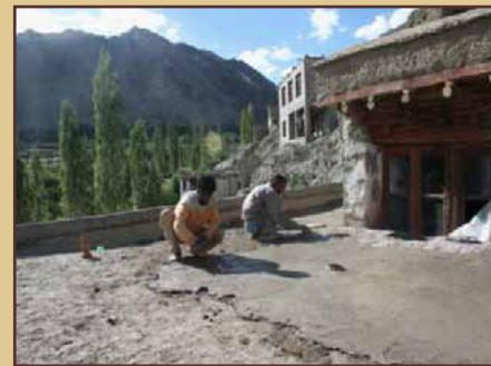
Load on the roof is reduced by removing additional layers added over the years. Proper drainage slopes and spouts were provided and the mud roof relaid
